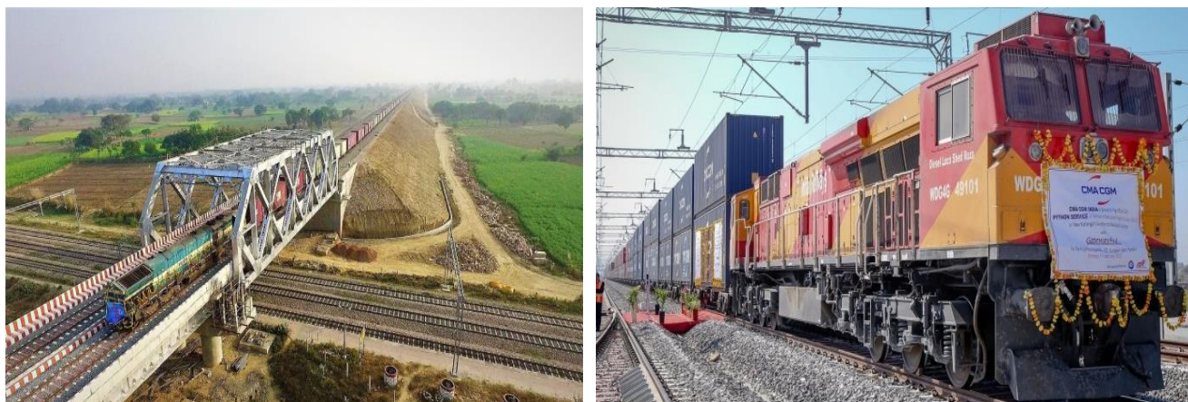
Dedicated Freight Corridor (DFC)
